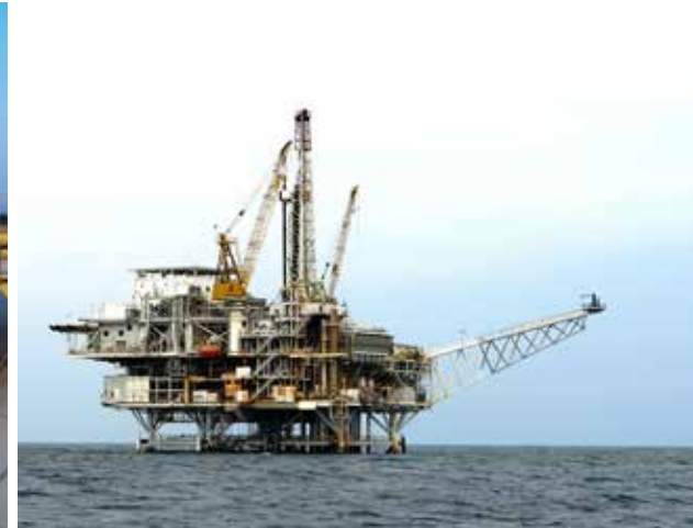
Solutions are tested before being commissioned
